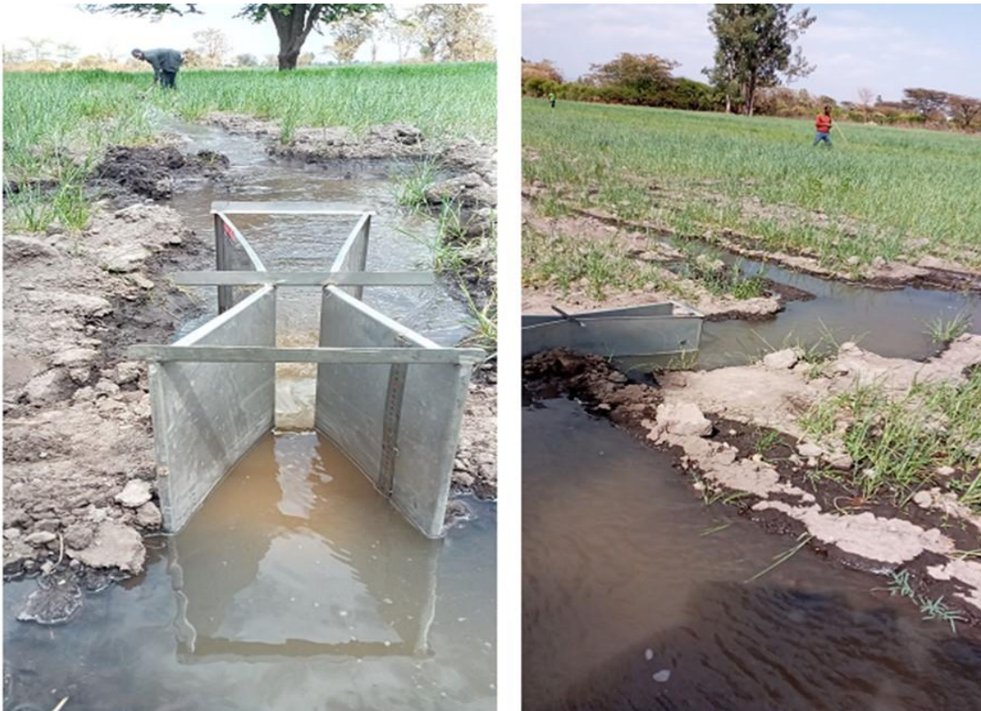
Figure 3.3: Measuring the irrigation water depth using the cutthroat flume
